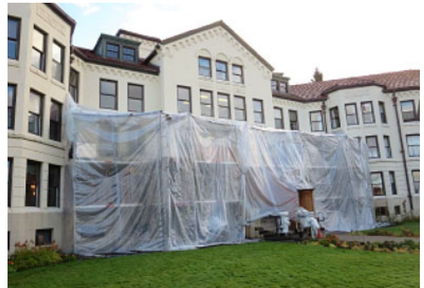
Refurbishment of the main entrance is completed.
